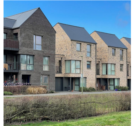
Barton Park, Oxford. Marker buildings adopt an altered roof and materials.
