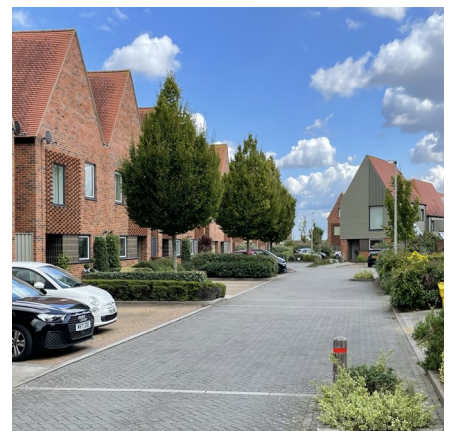
Horsted Park, Chatham. Marker buildings demarcate the end of a vista, with an alteration in architectural detailing and material palette.
