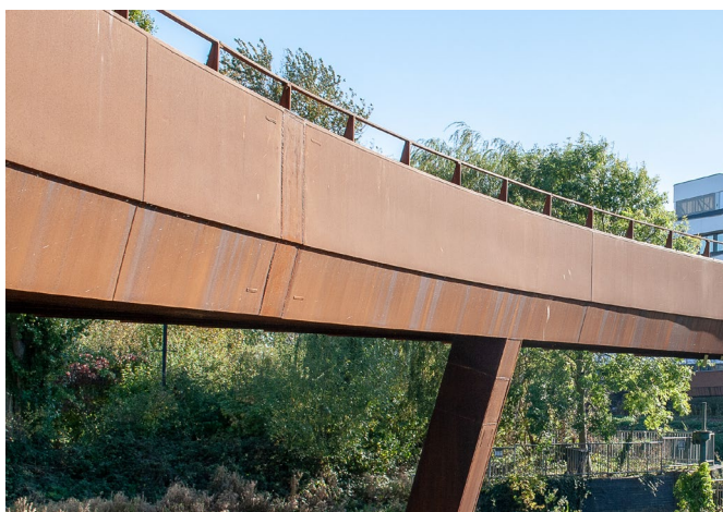
Active Travel Bridge in Northampton.
